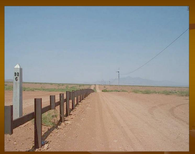
The heights of the posts are now staggered to prevent ramps from being set up to allow vehicles to drive over.
