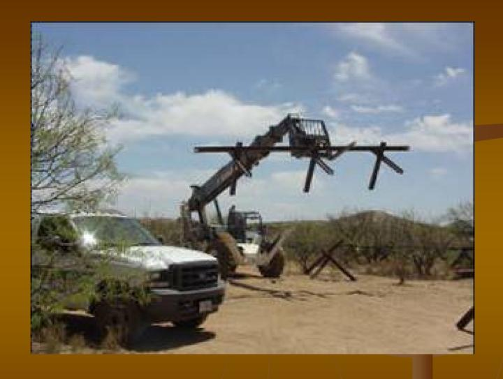
Temporary Vehicle Barriers can easily be installed with minimal ground disturbance to sensitive areas.
